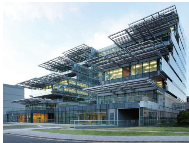
Slika 2. SIEEB Solar Energy-Efficient Building u Peking
