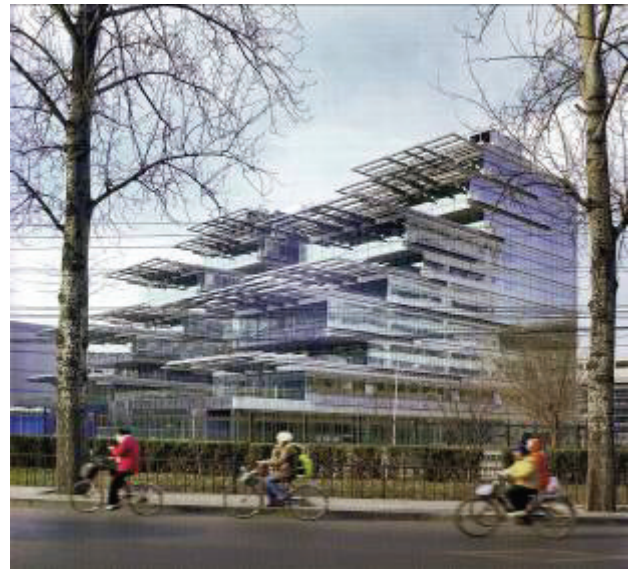
Sl. 2. Zgrada SIEEB (Sino-Italian Ecological and Energy Efficient Building) u Pekingu, Kina
